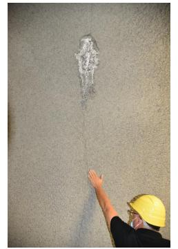
Figure 4: Crack and wet spot in Cavern 1 [Master Builders Solutions]
