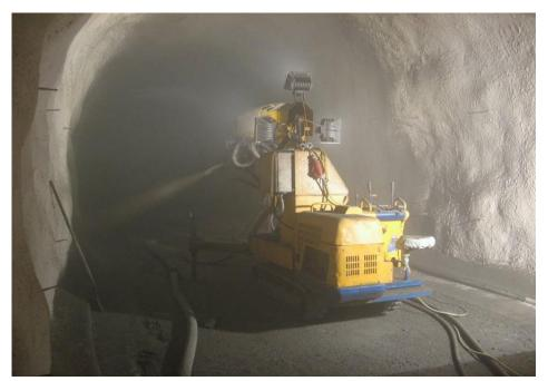
Figure 3: Application of the final sprayed concrete layer [Master Builders Solutions]
