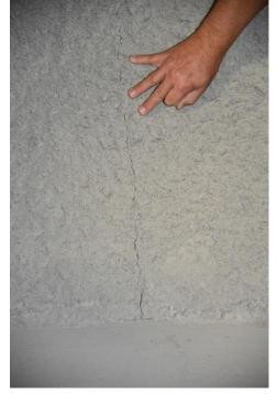
Figure 5: Crack from invert upwards (here Cavern 3) [Master Builders Solutions]
