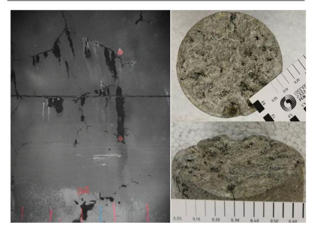
Figure 5: Left photo: Cracking of sprayed concrete visible as dark lines from water ingress, in rock support sprayed concrete in the research section of the Ulvin access tunnel. The red lines in the lower part indicate 1 m spacing. Right: Detailed crack images showing the use of a crack measuring gauge on a sprayed concrete sample from the rock support lining in the Gevingås rail tunnel. The core diameter is 76 mm [1]
