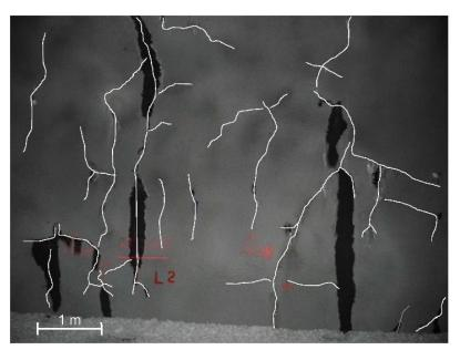
Figure 4a: Mapping and assessment of in-situ cracking of rock support sprayed concrete in hard rock. Observed and measured cracks are highlighted with white lines. Example from the monitoring and research section of the Gevingås railroad tunnel, Norway [1]
